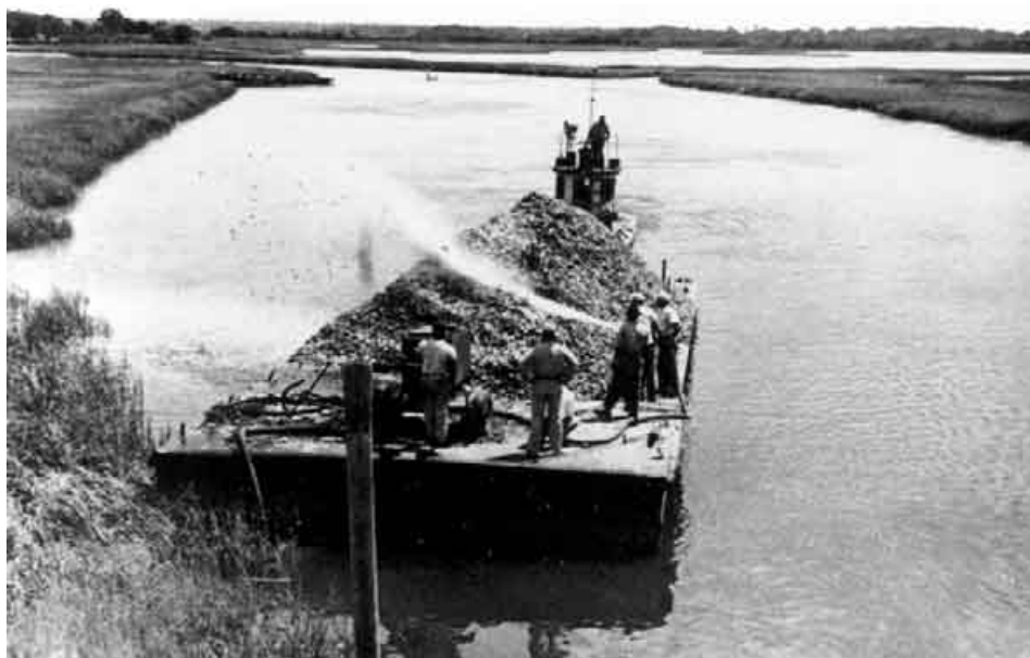
Figure 31. Washing shell onto intertidal beds with a water cannon in 1952 (Lunz Collection, Charleston Museum).
