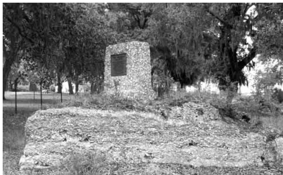
Figure 4. The remains of Fort Frederick at Beaufort, S.C. This was one of the largest “Tabby” forts. Built 1735-58 (Burrell photo).
